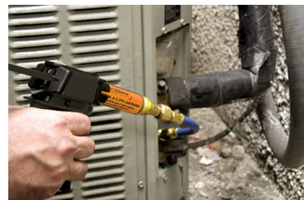
Step 3: Inject, then discard empty cartridge.
