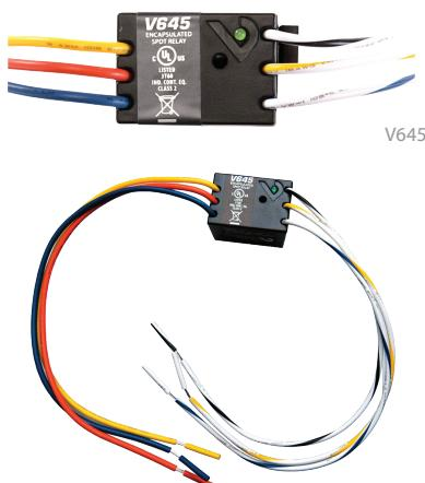
The Victory 645 is an economical, multi-purpose relay designed for control of loads up to 10 A. Its small size allows for space saving utility in panels and field enclosures.
