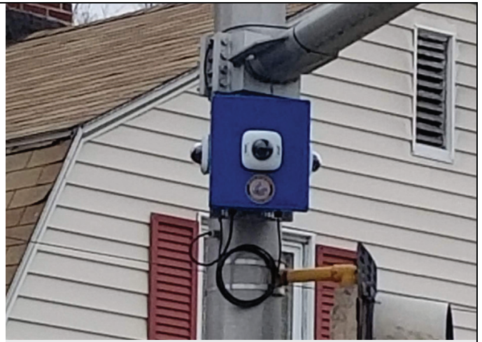
The FLIR Ariel Full HD Mini-Dome camera delivers high-resolution, clear video, even in high-motion or lowlight scenes.
