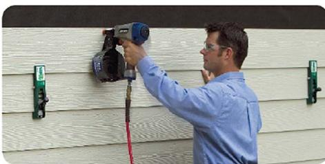
**4** Nail siding per manufacturer's recommendations. Remove both gauges and repeat steps 1 through 4 as you work upward to top of wall.
