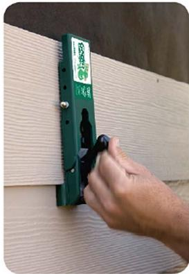
**2** Engage the handle for a snug fit. **Don't over-tighten!** (See photos A & B)
