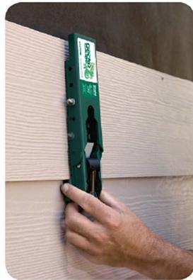
**1** At approximately one-third of your siding's overall length from either end, place the Gecko's blade under bottom edge of siding and slide upward.
