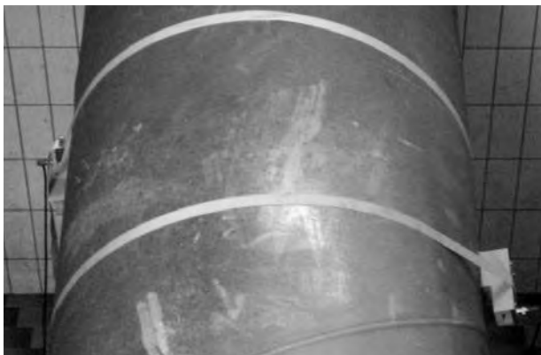
FIGURE 44: Z-mode installation with fabric-reinforced tensioning tapes for large pipe diameters
