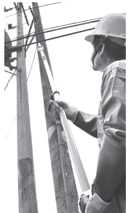
Fig. 3: Voltage detection for overhead lines
