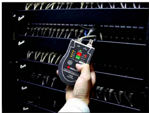
Confirm continuity and fault type
