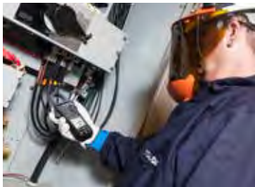
Analyze Power-related Issues
