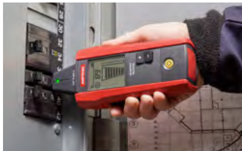
Identify the single correct breaker
