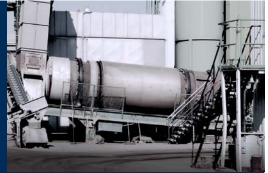
Application example: rotary kiln in the chemical industry
