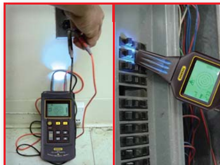
Locating a circuit breaker
