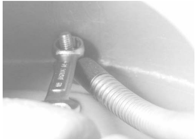
Figure 14 – Removing Pigtail Anchoring Bolt
