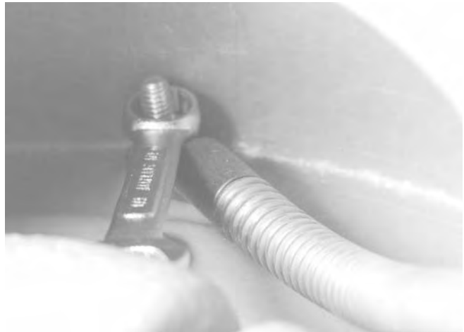
Figure 14 – Removing Pigtail Anchoring Bolt
