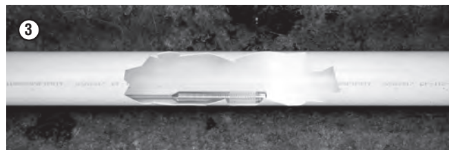
RE-INSPECT THE LINE TO ENSURE IT IS FREE OF DEBRIS AND CONFIRM LOCATION AND SIZE OF REPAIR
