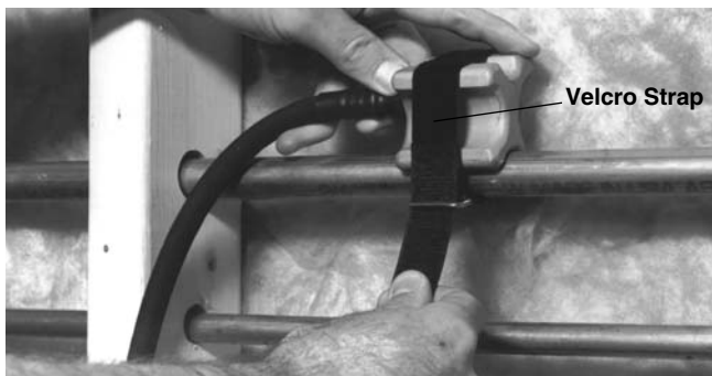
Figure 5 – Applying Freeze Head with Velcro Strap
