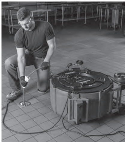
Figure 9 – Lubrification de la gaine de câble
