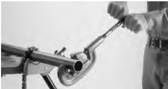
Figure 1 – Cutting End of Pipe
