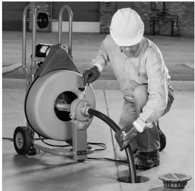
Figure 15 – Using Machine with Guide Hose
