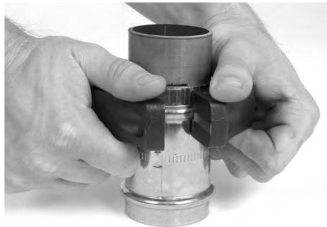
Figure 8 – Installing Press Ring Onto Fitting
