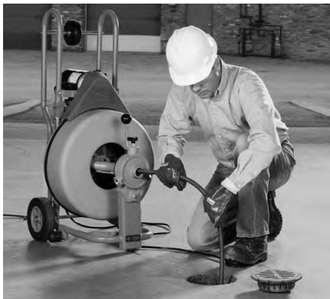
Figure 12 – In Operating Position, Manually Feeding Cable
