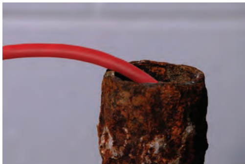
Figure 16 – Avoid Pulling at Sharp Angles
