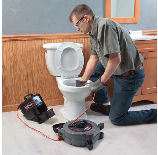
Figure 14 – Performing an Inspection
