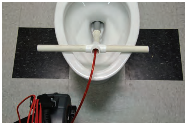
Figure 23 – Using a PVC Guide Tube
