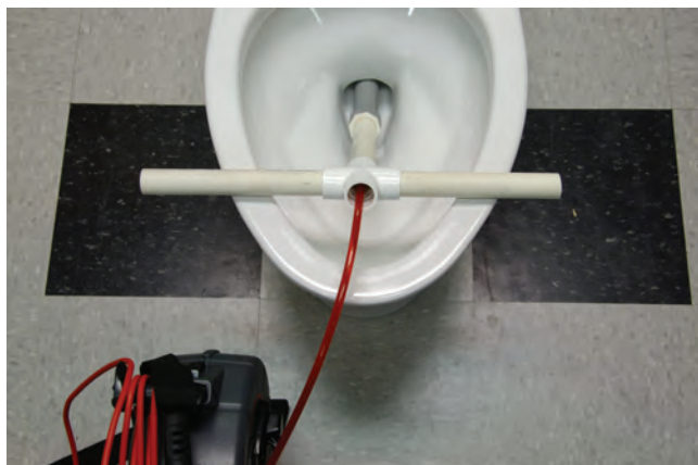
Figure 23 – Using a PVC Guide Tube
