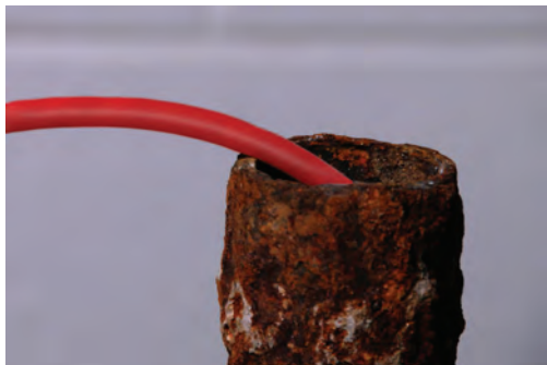
Figure 16 – Avoid Pulling at Sharp Angles
