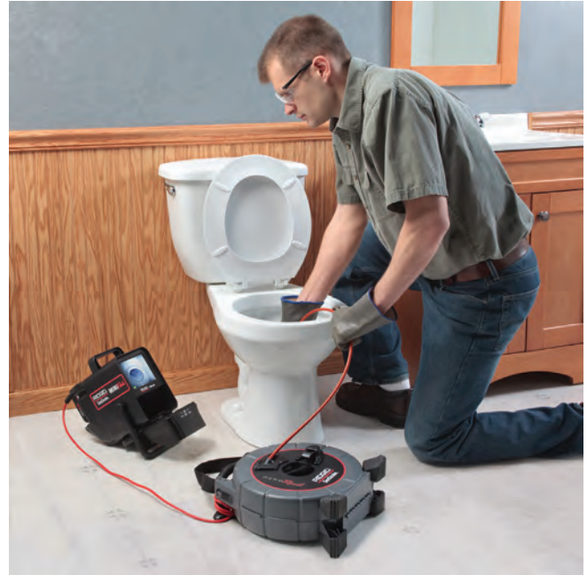
Figure 14 – Performing an Inspection
