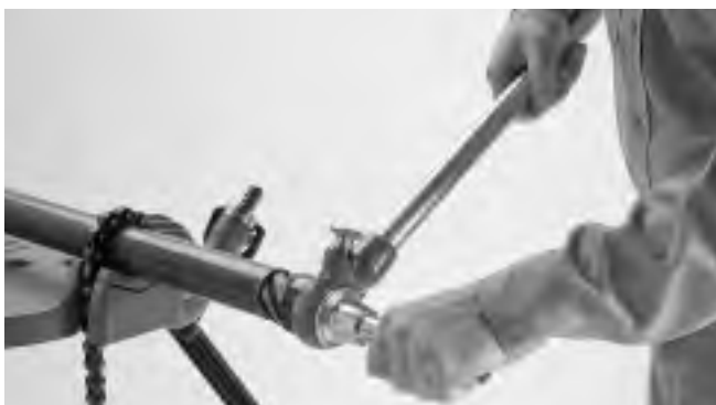
Figure 2 – Reaming End of Pipe
