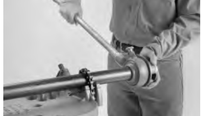
Figure 3 – Sliding Threader On Pipe
