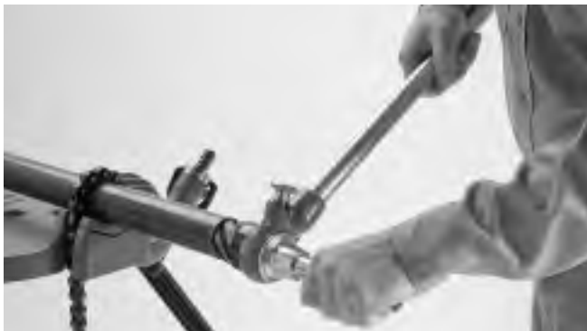
Figure 2 – Reaming End of Pipe
