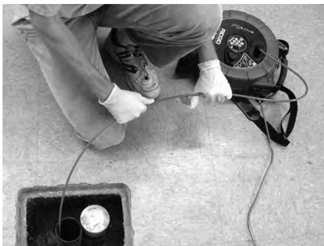
Figure 29 – Allowing cable to loop may kink the cable while pushing into drum
