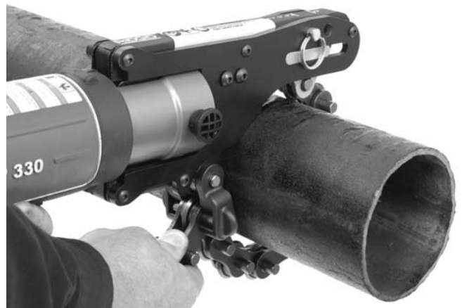
Figure 4 – Wrapping Chain Around Pipe
