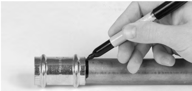
Figure 8 – Marking the Tubing After Fully Inserting Tube
