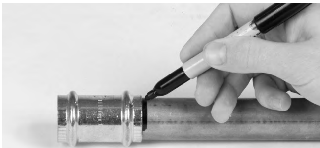
Figure 8 – Marking the Tubing After Fully Inserting Tube
