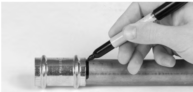
Figure 8 – Marking the Tubing After Fully Inserting Tube
