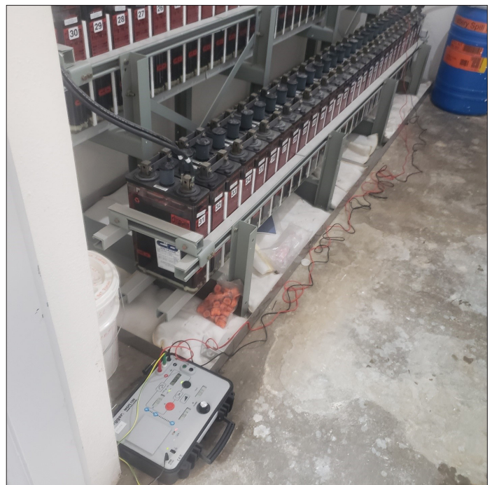
Figure 1: the Megger MGFL confirming a negative ground fault on the battery string
